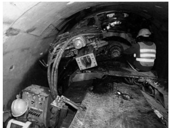
Fig. 4 Pilot Drilling on TBM (Kruppe HB-40A)
